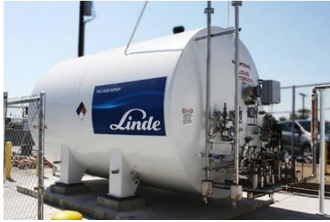
Figure 5 Cryogenic storage tank (left), gaseous storage supply (right) [9]
