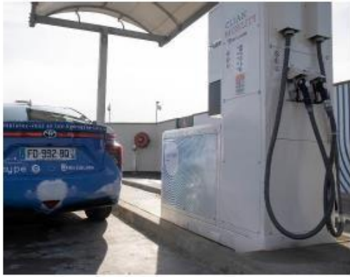
Figure 12 Dual dispenser for LDV refueling (left), scheme of refueling interface (right) [7]
